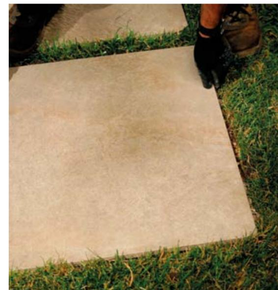
Aextra20 can be easily installed onto grass substrates simply by following the recommendations set out here: trace the encumbrance of the slabs and dig the substrate up to 3 cm. Then apply a layer of gravel to ensure perfect drainage and proceed with the installation of slabs always checking the planarity of the surface.
