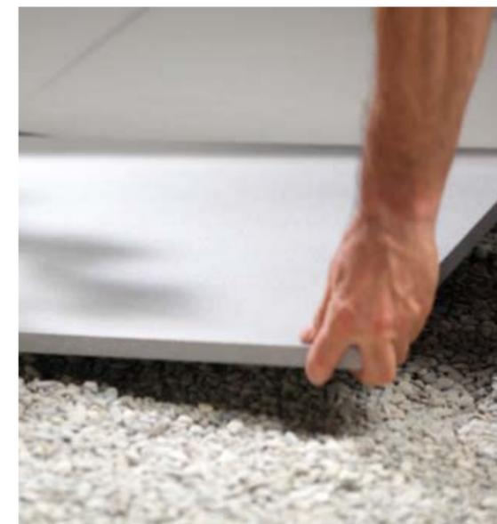
Aextra20 can be installed onto gravel substrates simply by placing the slabs adjacent to one another or creating pathways by installing individual slabs onto the gravel support. It is also advantageous to integrate, below the layer of superficial gravel, another layer of gravel and or pebbles in order to ensure perfect drainage. This installation solution is functional, quick and with a strong visual impact.
